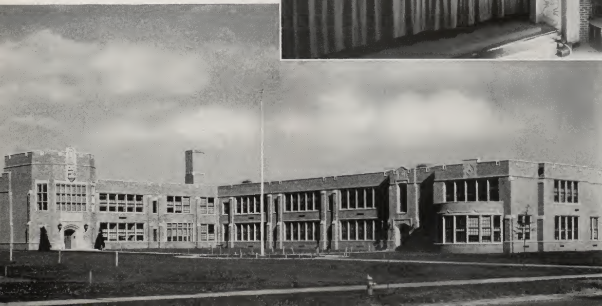
Stewart Avenue Elementary School, Garden City, Long Island—another firesafe school economically erected with lightweight concrete masonry backup and partitions. Architects, Tooker & Marsh. Builder, John H. Eisele Company.
